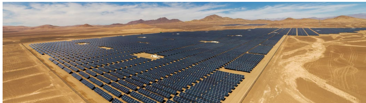
The Chañares plant in Chile has an installed capacity of 40 MW and can generate up to 94 GWh per year. © Enel Group
